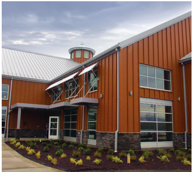
Port of Kalamazoo Interpretive Center, Kalamazoo WA (Weathered Zinc - Standing Seam Roof and Burnt Rust - Wall Cladding)
