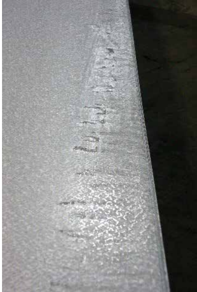
Light corrosion on stacked flatsheets.
